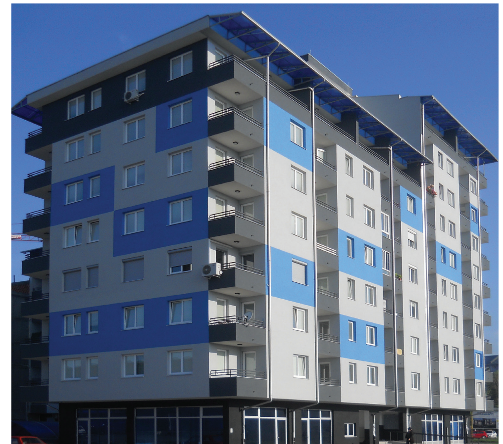
Residential building, Doboj
